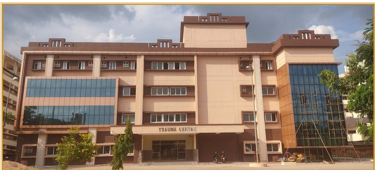
New Trauma Centre building
